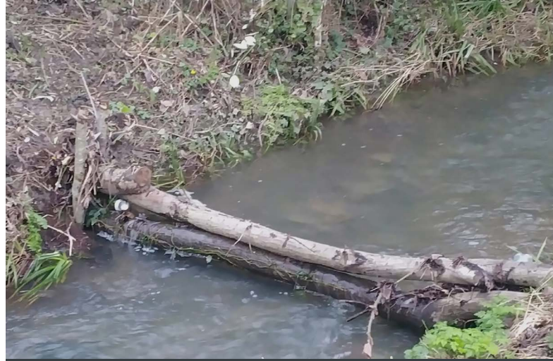
Plate 4 Pigeonhouse Stream Leaky Dam
